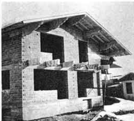
Concrete block home under construction, showing details of beam application. Finish surface is white stucco and brown stain.
