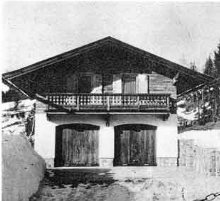
A two-car garage occupies the lower level of this modern Alpine design, and the arched openings are adapted for this purpose. It represents an excellent application of traditional elements to modern requirements.
